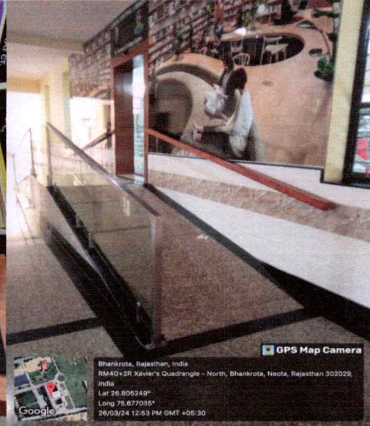
Ramp and Railing for Easy Access to Library
